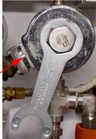
Figure 61. Remove nut from back of valve
